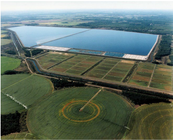
Muskegon County Wastewater Treatment Plant
